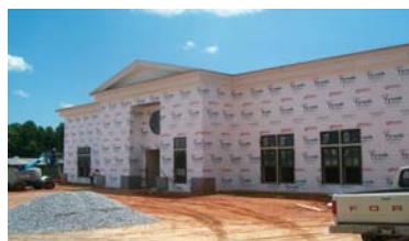
Main Drive and Entrance
